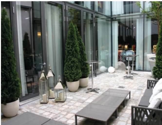
Ground-level glass wall made of IGU from tempered glass
