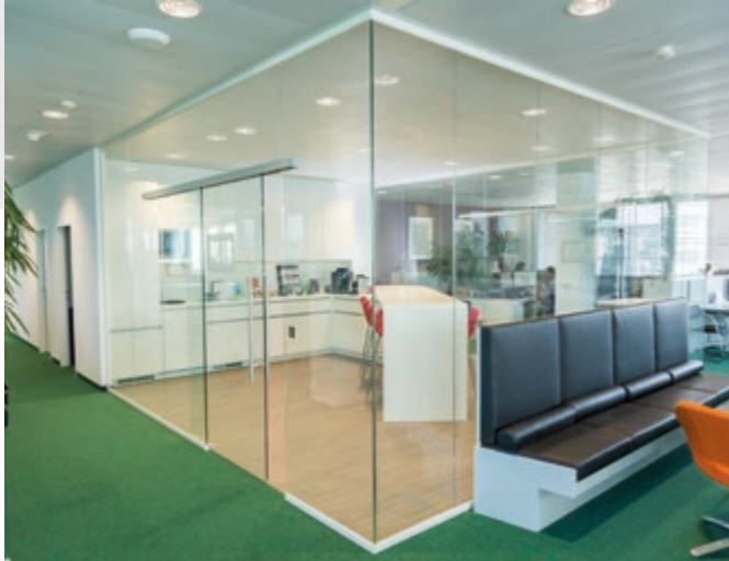
See-through room partition made of tempered glass
