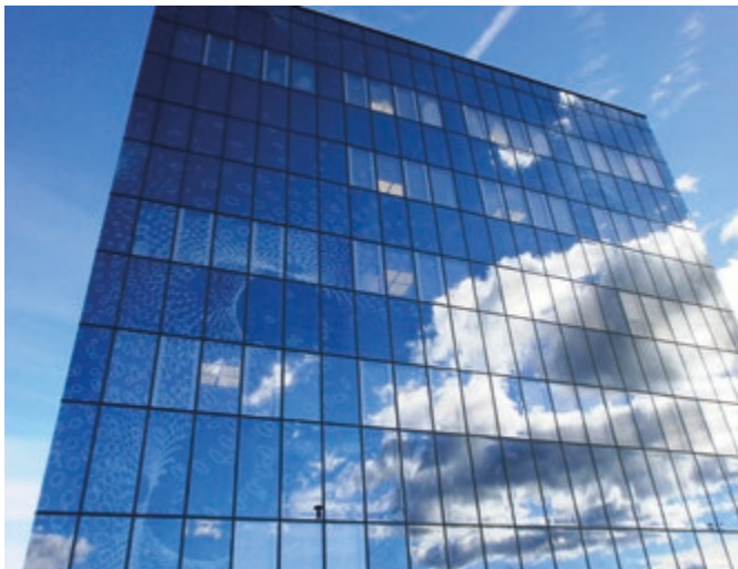
Curtain façade made of heat-soak tested tempered glass with design print
