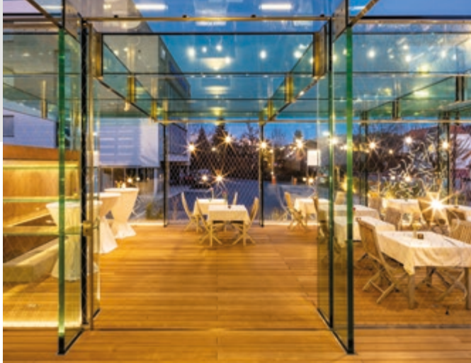
Glass beams with load-bearing function
