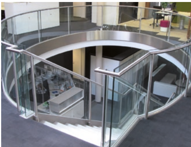
Glass balustrade clamped on one side only
